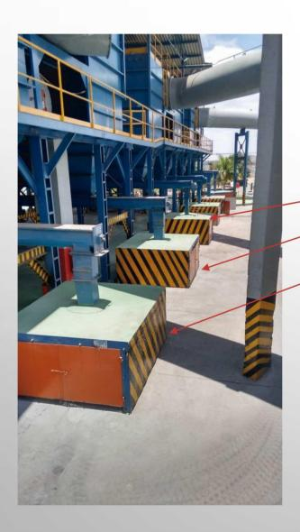
Laborious process to take the dust from the bag filters deposited in those containers and transporting by forklift to the shed
